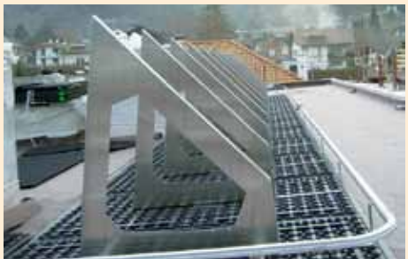
Linking the system with aluminium profiles, for example in a wind zone 2 location, with the adjunct "coast" and unfavourable structural conditions.
