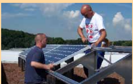
The solar panels are installed.
