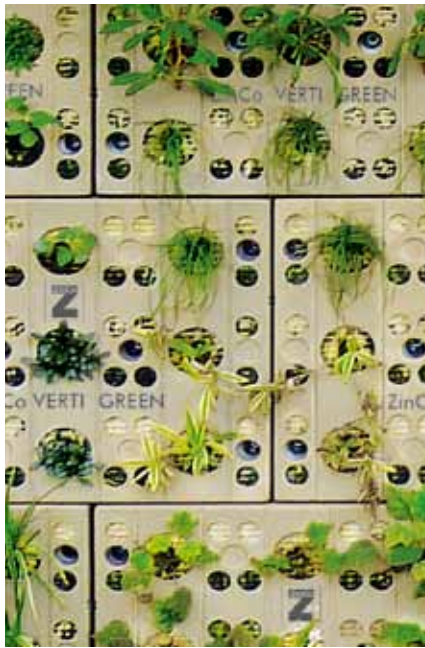
Modules immediately after installation
