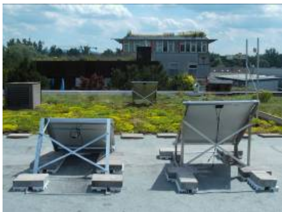
File name: ZinCo-Hallenvordach_Solar.jpg
