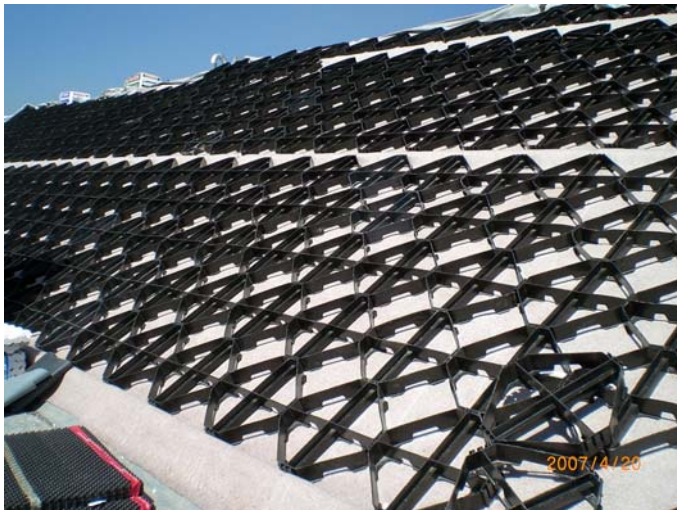
Image 5: The ZinCo-Georaster®-elements applied over the full surface provides reinforcement for the subsequently applied substrate layer
