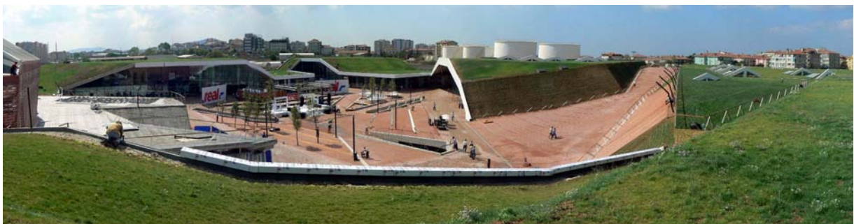
Image 3: The Meydan complex of buildings after completion of the green roof installation
