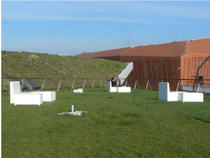
Image 10: Garden furniture placed on the accessible roof areas invite you to linger.
