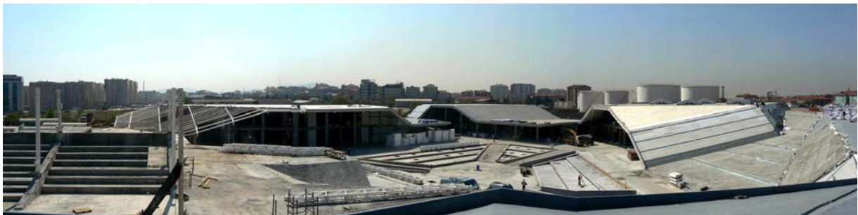
Image 2: An overview of the construction site before the green roof installation starts
