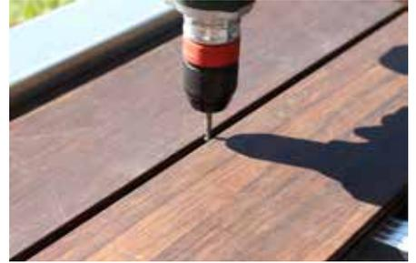
Generally, the fixing elements can be easily screwed into the rails and are invisible.
