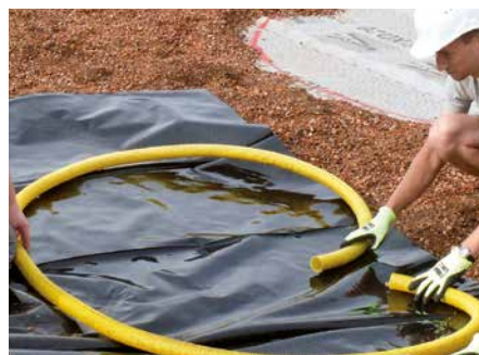
Temporary water bodies are created using drainage pipes and sheeting.
