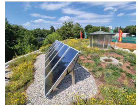
The green roof was combined with the existing solar energy unit – therefore producing synergy effects.
