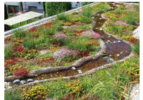
Insects and birds need water areas: They can be installed on the roof with sheeting.
