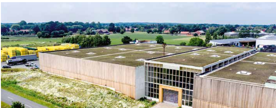
The 10,000 m 2 large green roof was created in collaboration with Osnabrueck UAS with biodiversity typical for the region on the warehouse roof at Luetvogt. © Architekturfotografie Steffen Spitzner
