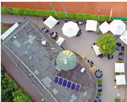
The KETV roof as a “naked” bituminous roof prior to the re-design as a green roof.
