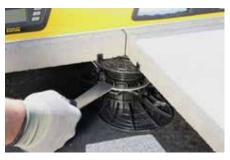
The new adjusting tool allows for the easy and subsequent adjustment and accurate setting of the required height, even after the pavers have been laid.
