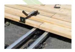
Given the flexibility of the rail system, it is easy to deal with the required decking lengths, in order to retain a stable butt joint for the decking elements.
