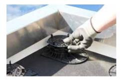
The oval shape of the new Elefeet® base plate enables the pedestal to be placed right at the roof edge and, once a cut has been made along the pre-defined line, even directly in the corners.
