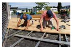
The wood decking can be easily and quickly fixed to the rail system with little effort.
