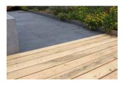
The transition between different types of walkway are easy to execute with Elefeet® pedestals and the Elefeet® Support Rail System,and are stable and sustainable.
