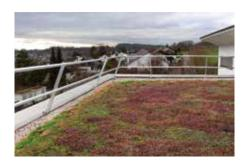
A collective fall protection solution such as Fallnet® ASG has the advantage that each person working on the roof is at the same time protected from falling off the roof. The ASG Maintenance Guardrail can be installed either vertically or at an angle. The Fallnet® ASG is Dekra-certified.
