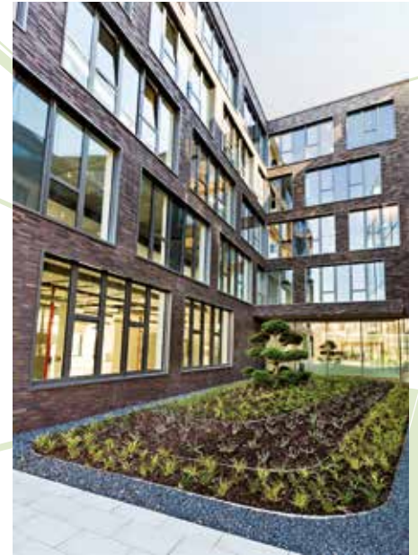
Inner courtyard equipped with a Stormwater Management Roof build-up on top of an underground car park in Ratingen, Germany.
