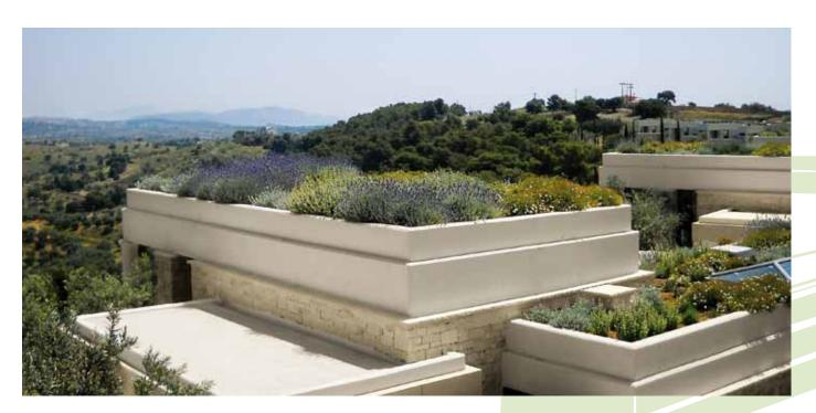
The semi-intensive system build-up "Heather with Lavender" allows for sophisticated planting design. Nevertheless, compared to intensive green roof build-ups, it manages with relatively low maintenance and relatively low build-up heights.
