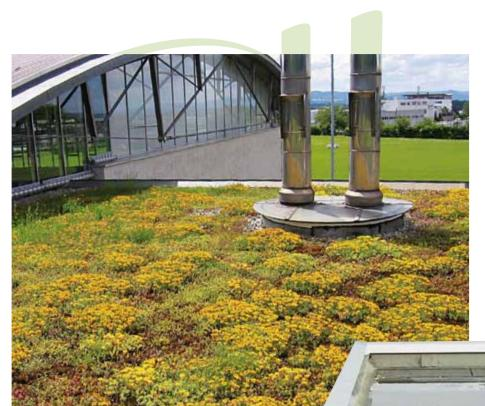
On 0°-roofs where deeper puddles might remain, the standard extensive system build-up is to be modified.
