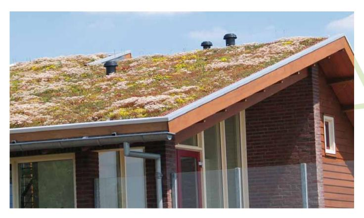
In general, flat roofs should have a slope of at least 2 %. Pitched roofs, as described in this brochure, start with a slope of 10° (18 %). From 10° on, the Green Roof system build-up differs significantly from system build-ups below 10°. Shear forces increase with the roof slope and have to be transfered into stable beams. The substrate layer has to be protected against erosion.
