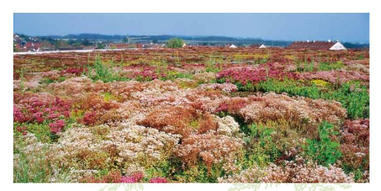
The "Sedum Carpet" is a standard build-up for extensive Green Roofs. It is a shallow and lightweight Green Roof type with an attractive "back-to-nature" appearance, that requires little maintenance.
