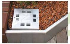
An inspection chamber incorporated into the system build-up
