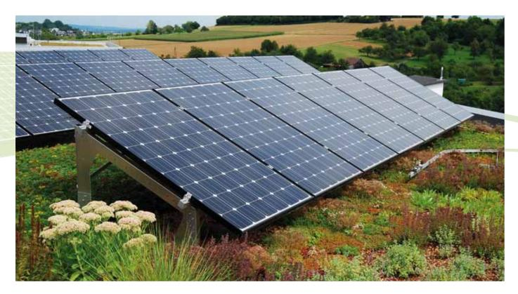
Green Roofs include a range of benefits. They can add thermal insulation, protect the waterproofing, improve biodiversity, retain storm water and improve the microclimate. ZinCo extends the advantages of Green Roof technology with the development of support bases for solar panels. With the innovative Solar Base, solar energy can be integrated into Green
