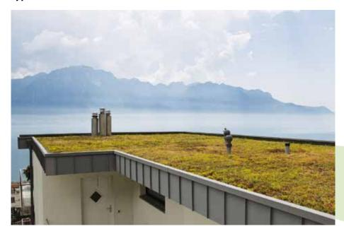
Extensive landscaped roofs are an ecological alternative to conventional surface protection or ballast layers such as gravel and pavers. They are lightweight and have a shallow build-up height. Suitable plants include various
