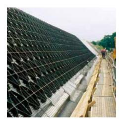
The system build-up "Steep Pitched Green Roof", based on the Georaster® elements, enables the installation of Green Roofs with slopes exceeding 20° and up to 35°. Above 35° special solutions can be designed by the ZinCo engineers.
