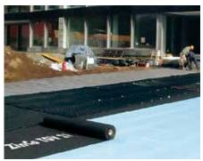
The characteristic of an inverted roof is that the insulation is above the water-proofing. The extruded polystyrene insulation (XPS) which is used for this kind of roof is impervious to water, but not to water vapour. Forming a vapour barrier directly above it when installing a Green Roof must therefore be avoided. Layers that prevent moisture from diffusing out mustn't be installed over the thermal insulating XPS boards and the layer above should be vapour permeable.
