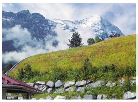
The plant selection has to be well adapted to the extreme conditions of Steep Pitched Green Roofs, where the solar radiation is the highest on the south facing roof side and the water run off is much faster than of a flat roof. The irrigation should be planned for, even if it is only needed in times of drought. It can avoid gaps in the vegetation coverage, which would lead
