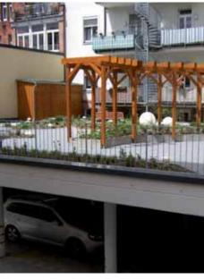
A pergola can be incorporated without penetrating the waterproofing, be it for additional plant support or simply as a design feature.
