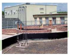
The boundary to the walkway has to be sufficiently high in the case of lush vegetation. Sandstone walls were used for this building in Frankfurt. The filled Floradrain ® FD 60 neo element proved to be the ideal basis for designing this leisure area at a lofty height.
