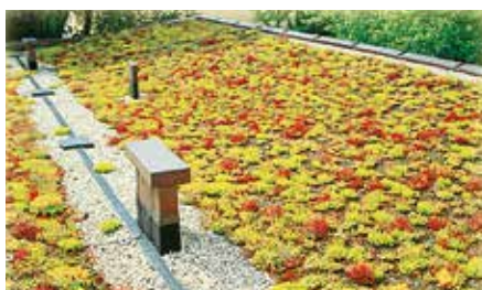
This roof with a pitch of approx. 5° is drained using a gutter and does not yet require any special measures.
