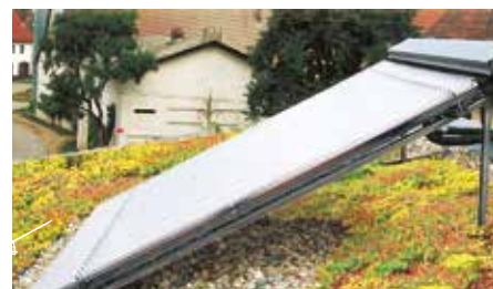
The use of solar energy is also possible on pitched green roofs. The issue as to how each system can be installed without penetrating the waterproofing, is addressed for each individual system.
