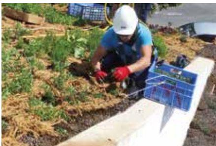
Finally, the roof is densely planted with various Sedum species and other perennials.
