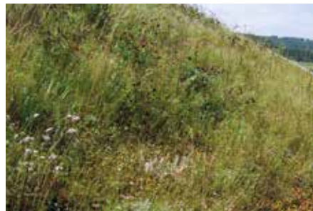
Even after only one vegetation period the plant coverage is largely complete. The roof area in this example is drained by means of an outer-lying gutter into which the three water spouts carry any excess water.
