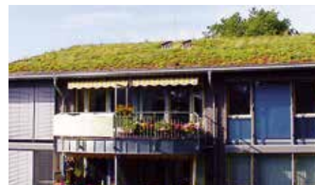
When determining the dimensions for eaves upstands or shear barriers, it is not only the saturated weight of the green roof build up that is relevant. Local snow loads must also be taken into consideration.
