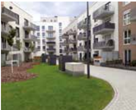
The planted and surface areas at Noltemeyer Hoefe conceal an impressive 5,780 m 2 of stormwater management area.
