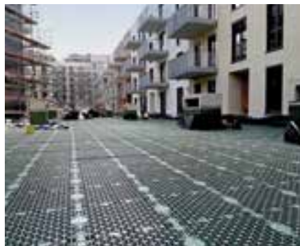
The fully installed stormwater management layer RSX 80 can store more than 75 l/m 2 of rainwater in its cavities.
