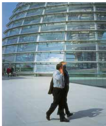
The combined protection and drainage layer, which has been applied here still protects the waterproofing membrane under the large scale concrete slabs.
