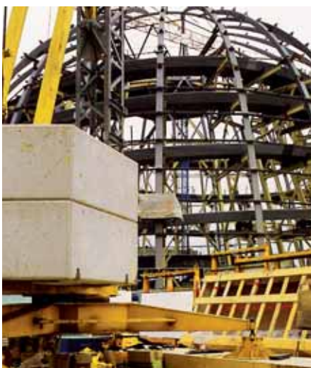
During the construction phase flat roofs are often used as storage space or place of constructions machines such as on the roof of the Reichstag in Berlin.
