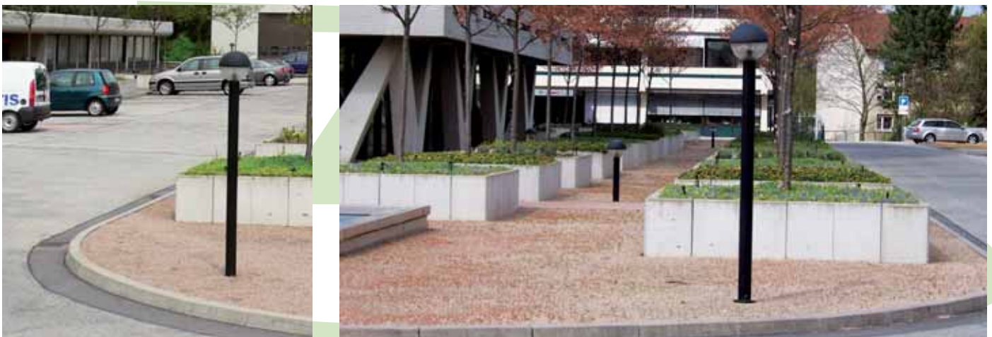
A continuous drainage layer based on Floradrain® FD 60 has been realized both below the planters and below the driveway.
