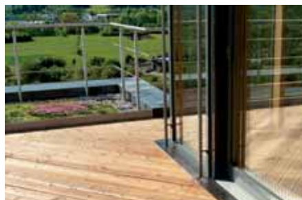
The design of thresholds is flexible as long as they correspond to the "Flat Roof Guidelines" or any relevant national regulations.
