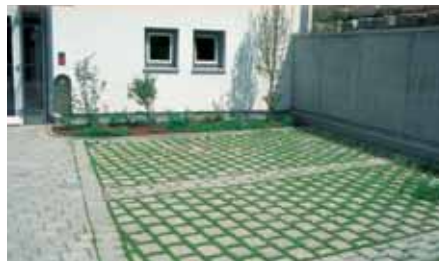
Pavement joint greening
